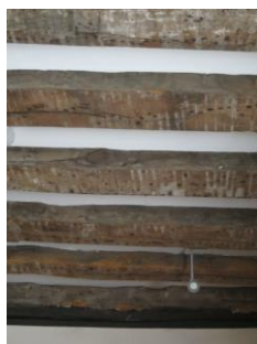
Floor joists of the first floor Hall
