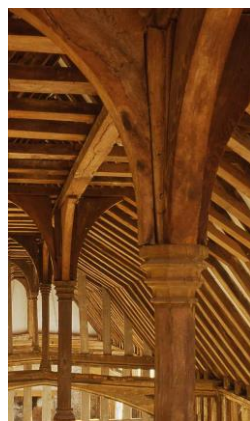
The crown post roof
