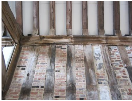
Studs with brick infill
